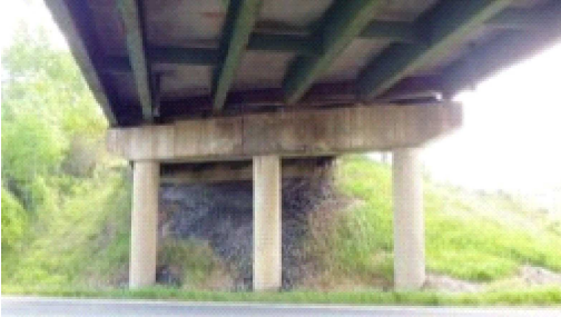
Existing pier at bridge #1
